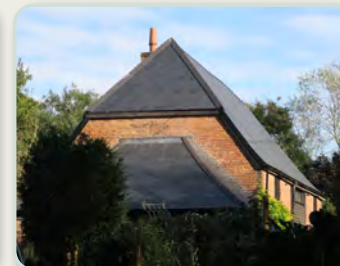
Half-hipped (jerkinhead) roof form with slate roof tiles
