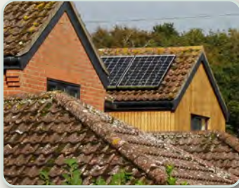
Norfolk stretcher bond red brick and timber weatherboarding
