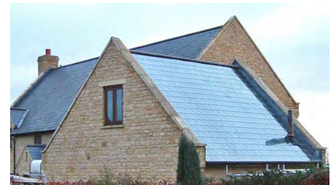
Figure 18: The placement of solar panels should be oriented for best solar gain. If these are visible from the street, they could use panels that resemble slate tiles.
