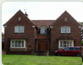
Cross-gable roof and double Gable (M-Gable) roof types
