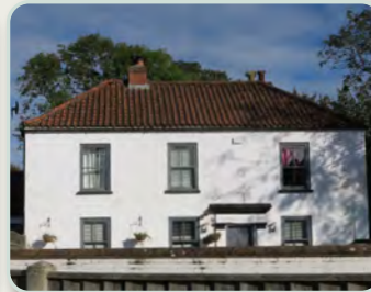
Hipped roof with concrete red pantiles and half barrel ridge tiles
