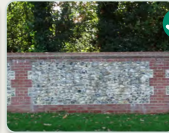
Uncoursed rubble masonry wall inset in red brick dressing
