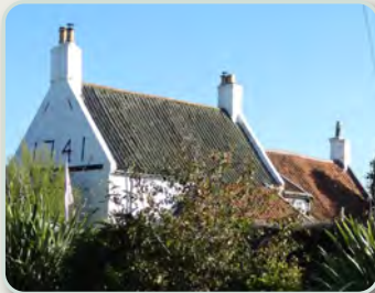
Gable end roof form with grey and red pantiles and ridge tiles
