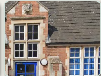
Stone detailing such as limestone lintels, panes, quoins and mullions
