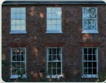
Sash windows with glazing bars and cills and brick, flared lintels
