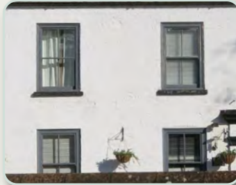
Windows are timber (painted here) and are flush with the facade
